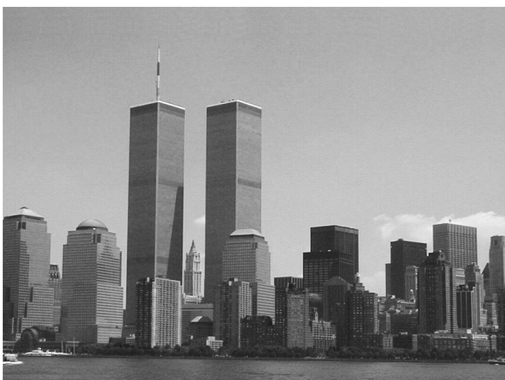
PICTURED ABOVE: Archival view of lower Manhattan. The World Trade Center buildings, popularly referred to as the Twin Towers, are visible in the foreground.
